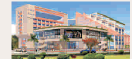
CITY CENTRE, Sansar Chand Road, Jaipur
