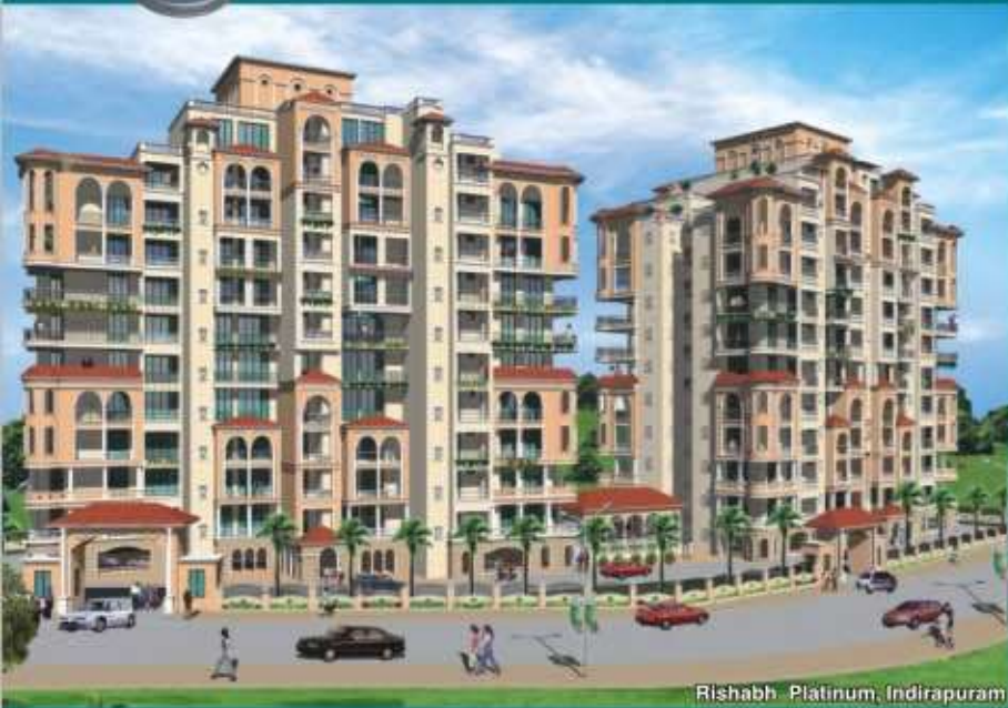
Rishabh Platinum, Indirapuram
